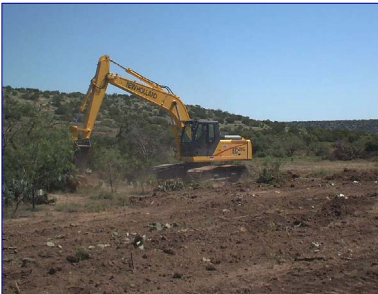
Grubber removing mesquite
