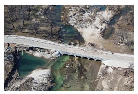
The devastating floods that hit Junction in October of 2018 did extensive damage to Flatrock Crossing on FM 2169. The crossing suffered damage to its bridge deck, buckling of pavement at the approaches, and the loss of the concrete sides of the approach to the bridge which were washed downstream with the torrential flow of water.
