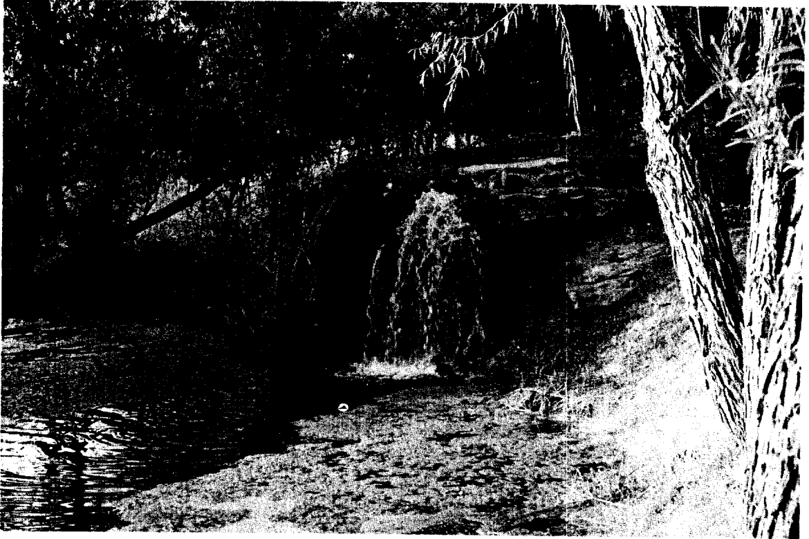
Figure 44.—Remains of Old Mill Dam at San Saba Springs
