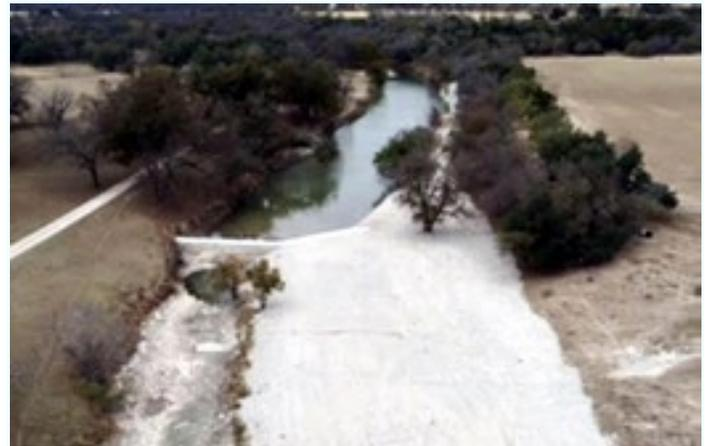
*Pedernales River dam: Note the built up caliche/gravel now heaped in the riverbed downstream of the dam that was dredged out of the riverbed upstream in order to deepen the pool created by the dam.*
